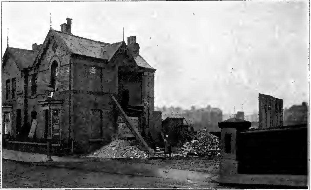
SCARBOROUGH: No. 2, WYKEHAM STREET, Where four people were killed.
